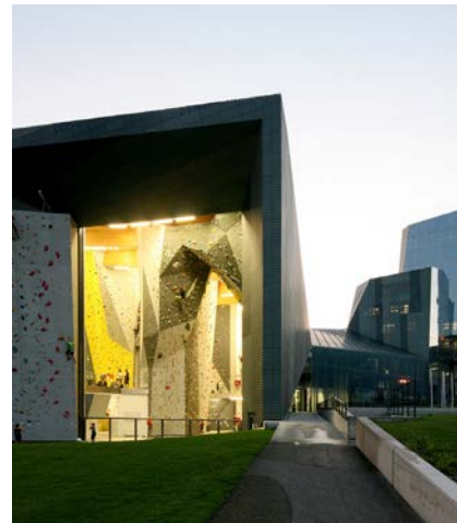
Salewa Headquarters, Bolzano/Italy (2007-2011)
