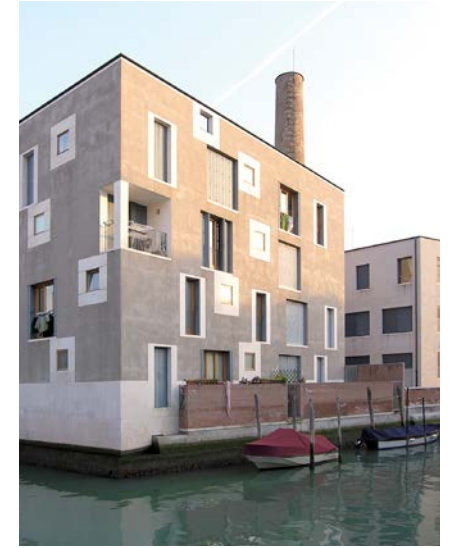
D Residential Building, Venezia/Italy (1997-2003)
